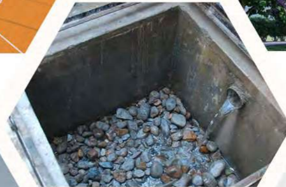
RAIN WATER HARVESTING
